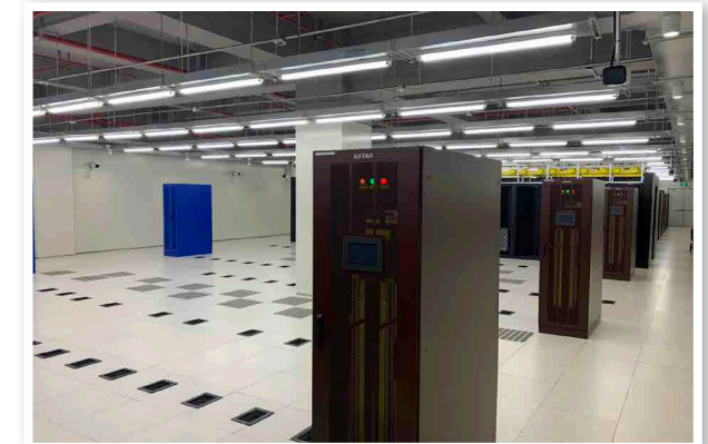
Some computer rooms of the Bank's Data Center adopt LED lighting sources, which can further reduce energy consumption
