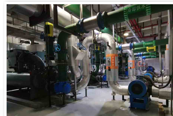
The Data Center's cold source station adopts color code management to improve equipment operation and management efficiency
