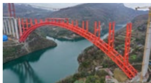
▲ Guizhou Branch of the Bank extended loans to support the construction of Wujiang Mega-bridge.
